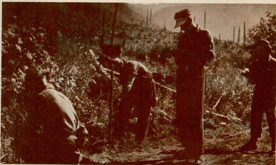
Surveying for a new road in Snoqualmie National Forest.
