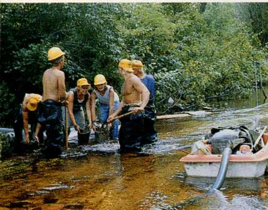
Foot by foot, YCC crews sandbag shallow streambanks to stem erosion, increase water flow and build better fishing habitat.
