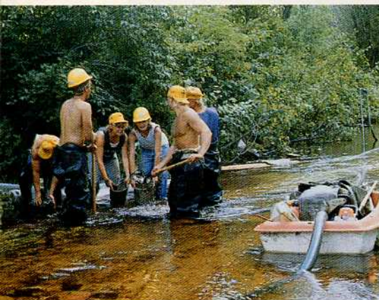
Foot by foot, YCC crews sandbag shallow streambanks to stem erosion, increase water flow and build better fishing habitat.
