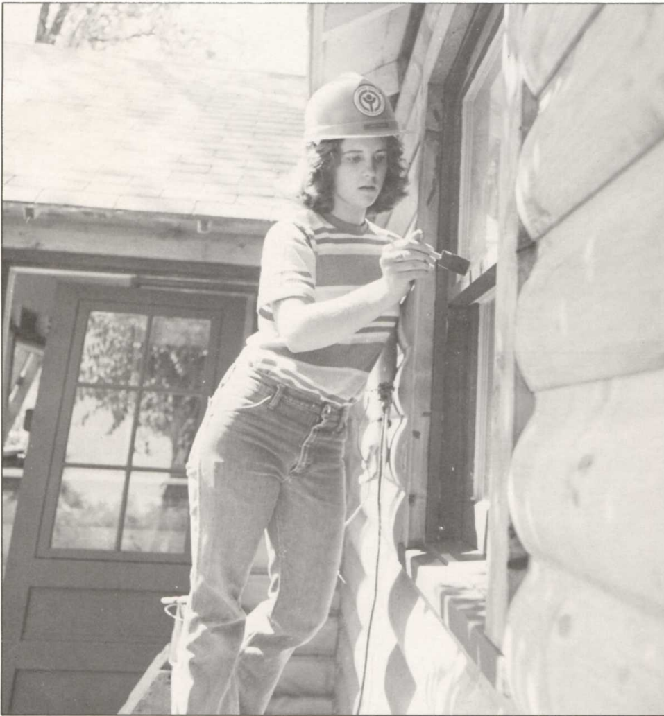
A YCC enrollee conducts cabin restoration work in Crawford, Nebraska.
